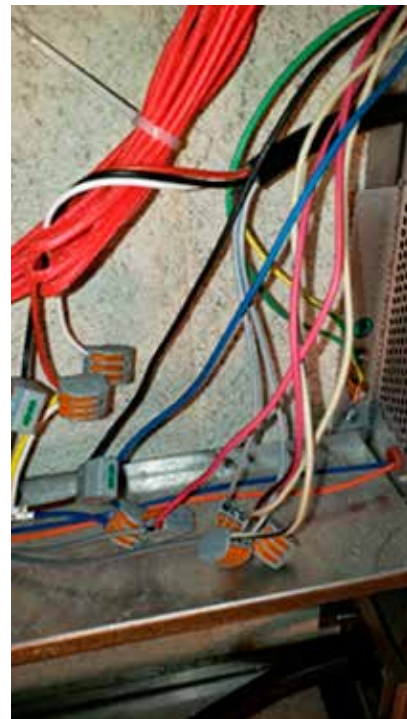
After Making Wiring Connections
